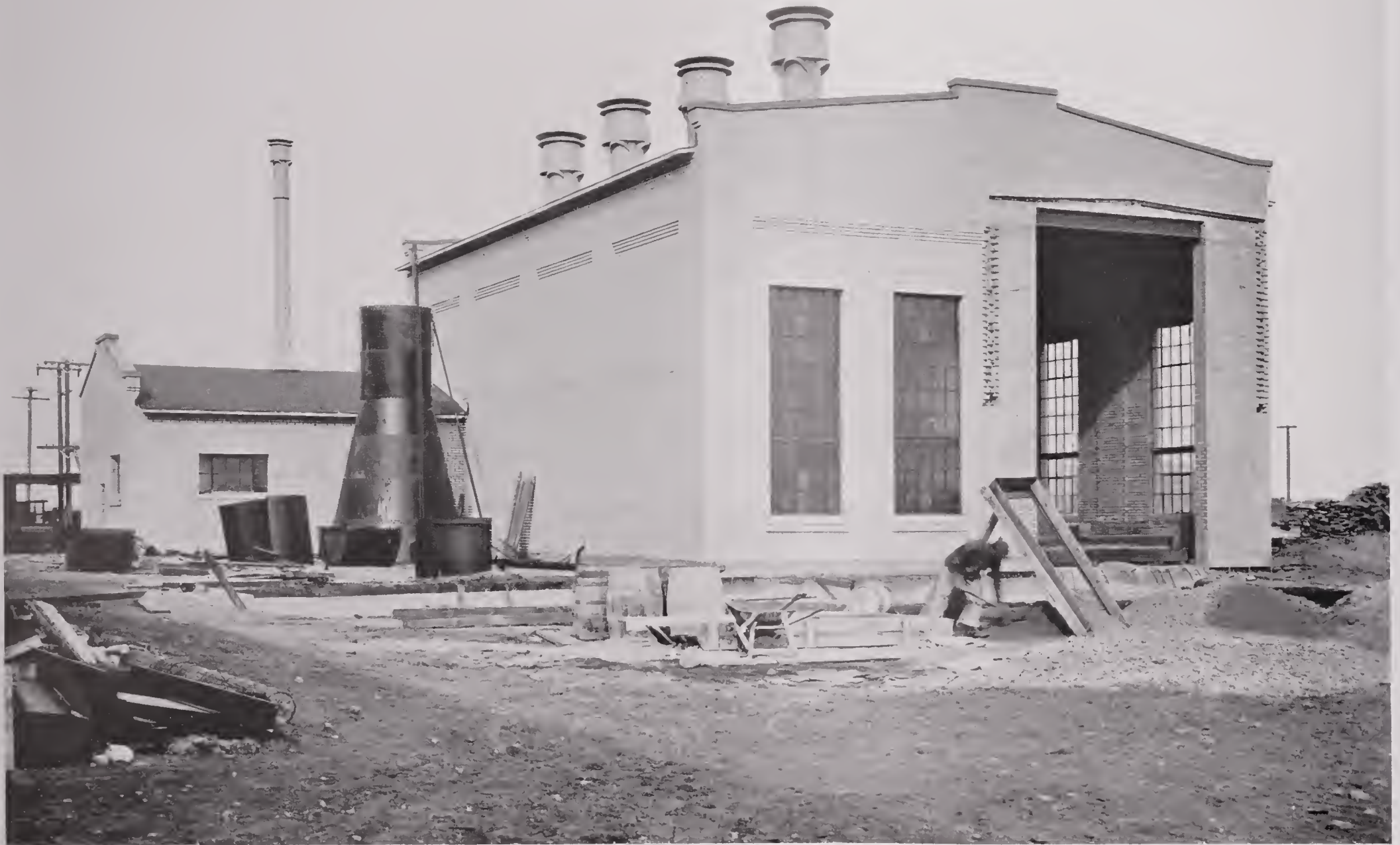
STEAM BOILER PLANT OF DROP FORGE DEPARTMENT
